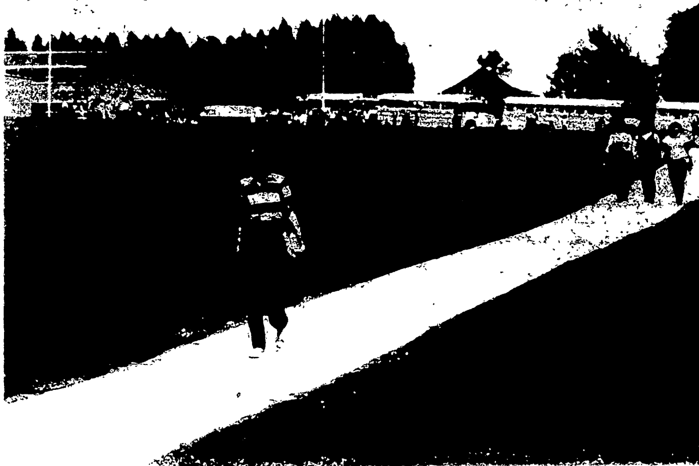
The new sidewalk from Manlius to the Fayetteville-Manlius High School is in place along Seneca Tnpk, giving FM pupils a way to walk to school without being in the highway. The walk was installed by Manlius Village workmen.
