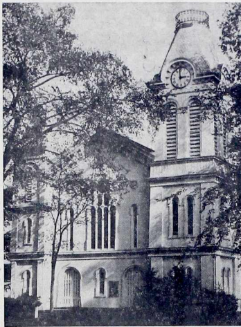
EAST HAMPTON'S First Presbyterian Church as it appeared before the recent remodeling job. Left above, and after the work was completed. The building was built in 1860, and then had the two steeples, one flat-topped.
